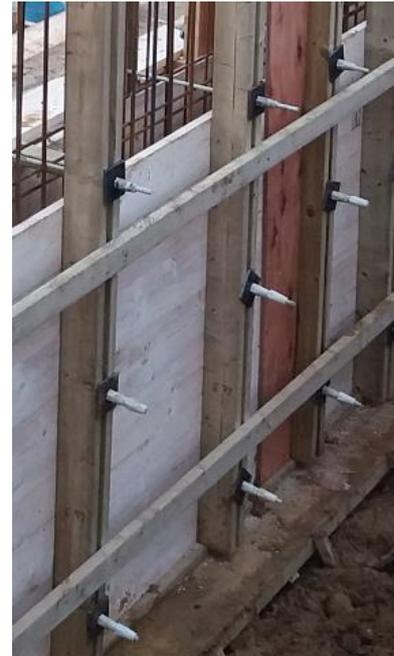
7. Rods can be cut and coupled together inside formwork with a full-size nut at any point. But the logic in '5' above applies. If near the bottom of a wall have 2 rods not one.
