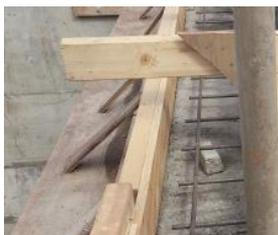
The traditional way of forming the edge of a podium deck requires a lot of timber - compared to a line of rods.
