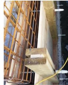
They are manufactured in China where their more usual use is in coal mines and as ground anchors. Throughout China new tunnels and steep sides are held up with a wire mesh held in place with these rods resin glued into the surrounding rock. A waler plate is held against the wire mesh with these nuts.
