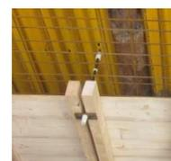
12. Where concrete is cast up against concrete piles or concrete underpinning, it is usual to hire in immensely strong (and no doubt expensive) single-sided shutters, such as this:
