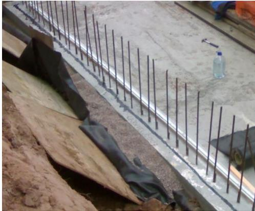
It might be considered easier to put the land drainage in before the walls are formed to provide something higher to stand on.
