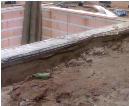
Wrapping the geotextile filter membrane over the top of the wall, tucking it behind and fixing it back with a screw strip through what is now 3 layers is preferable to a top cover strip that, because it is relatively rigid, suffers damage and fails far more readily, especially where it is trying to cover two sheets of drainage board overlapped at joints.
