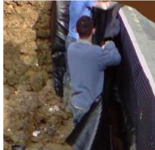
The drainage membrane will usually fold easily around external corners and into internal corners.
